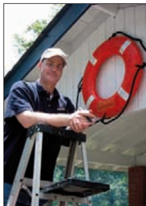
(Left) Sean Fennell installs a lifering to the AFRH pond pavillion.
