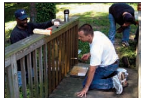
(Above) Staining the bridge.
